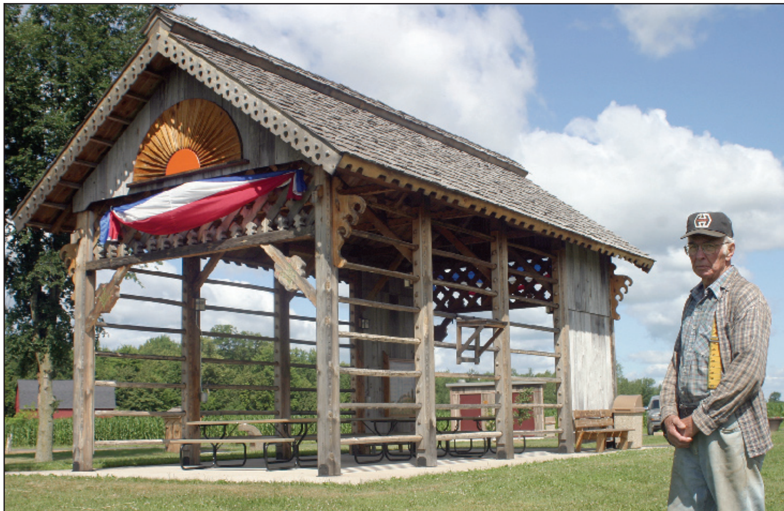
Bill Snedic stands near the kozolec he designed and built with volunteer help for the Willard Settlers' Park. The structure was used by Slovenian farmers in the old country for drying hay.
