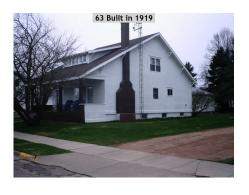
It is a large two story or what they call a 1 3/4 story wood frame home with stucco siding which is concrete over a heavy wire which is attached to the wood sheathing. Known as the Hiebsch House; the home is now owned and occupied by Robert and Diane Braun. The address is 167 North Front Street.
