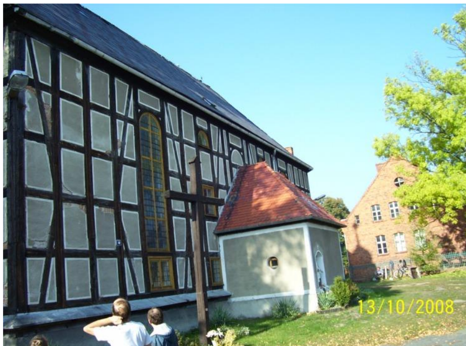
East side of the Kainowe Church (left) and former school (brick building on the right). According to the local priest, the exterior had been damaged by a fire around 1998.
